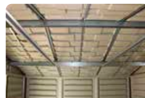
The wall columns, doors and roof are reinforced with solid metal support .
